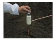
1 Insert the rod and conductor into the mould, locate the retaining disc and pour in the weld powder.
