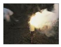
3 The resulting exothermic reaction reduces the weld powder to molten copper alloy which melts the retaining disc and flows into the weld cavity where it partially melts the conductors. The molten copper alloy cools to leave a fusion weld of great mechanical and electrical integrity.
