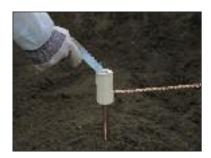
2 Place the lid on top of the mould, add starting powder and ignite with spark gun.
