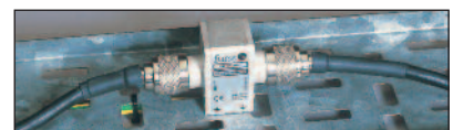
ESP RF 111121 on a coaxial cable running between an antenna and an RF receiver
