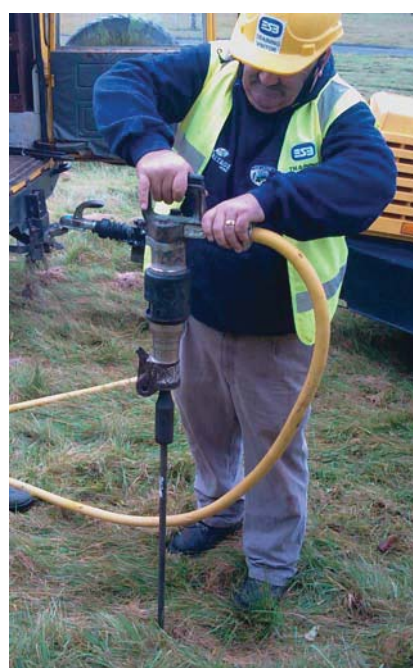
The driving down has started.
