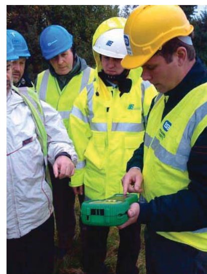
Measuring of earthing resistance.
