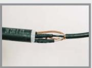
The outer insulation is then installed, and the core is drawn out in the same way as in the previous item and shrinks the hose immediately.
