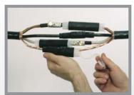
When the core is drawn out, the hose shrinks immediately and creates a safe insulation and moisture seal.
