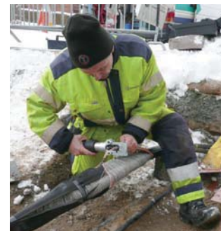
Crimping with Elpress crimp tool PVL611.
