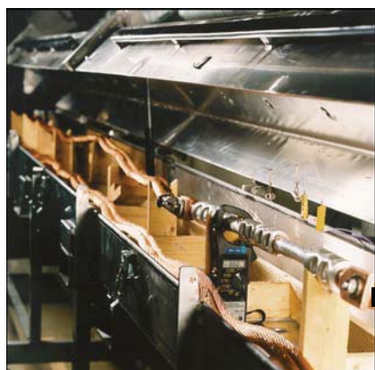
Testing of connections at the Elpress laboratory.
