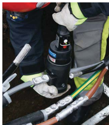
Crimping of Elpress Al through connector with crimp head V250.
